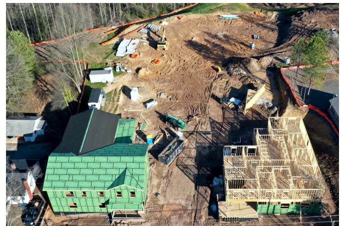
T-East homes being built
